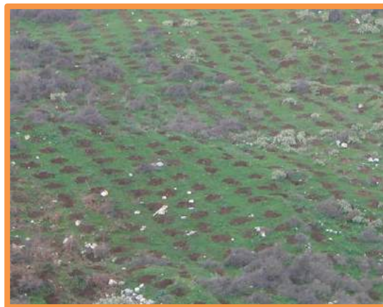
Figure 3.7. Hole excavation on flat terrain
